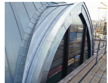
Kilgoot: handwerk (Foto: Ridder Skins for Buildings).
